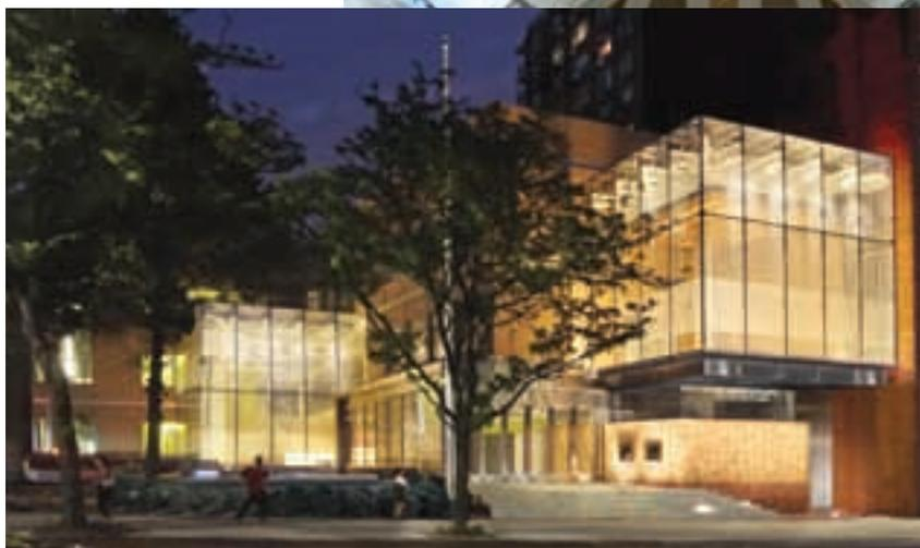
The boxes are constructed from heavy-duty Pilkington Optiwhite true low-iron insulating glass units with a low-coating, which reduces heat-loss from the space by reducing the amount of radiation of energy outwards from the building. Adding to the visual impact of the glazing, as well as helping reduce excessive heating and glare from the sun, is a white, silk-screened frit of vertical lines.
