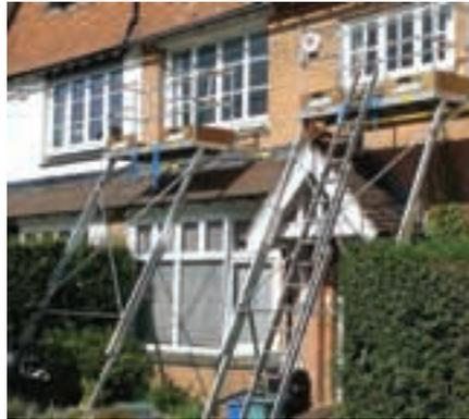
Easi-Dec Roofline is a modular system incorporating one or more Easi-Dec platforms linked securely with Easi-Dec Catwalk to form a continuous fully-guarded platform. It has been designed to provide simple, rapid access to roofline level by eliminating the time constraints of erecting scaffolding and can be set up in less than 30 minutes. □
